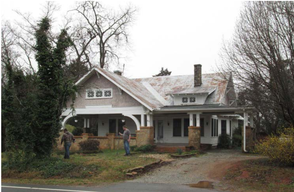
This house on Peeksville Road shows many characteristics typical of the Craftsman style, including square column porch supports, bracketed eaves in the front-facing gable, and a deep porch overhang.
