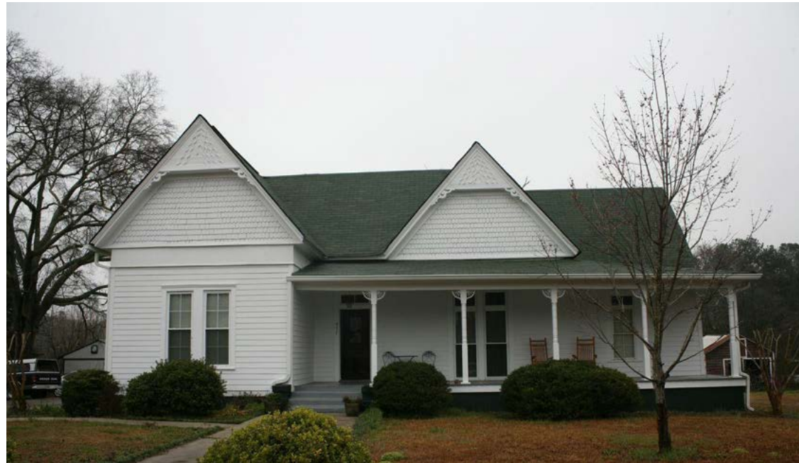
Some Folk Victorian details on this simple house form include the decorative eave trim in the front-facing gables and spindle work at the top of the porch supports.
