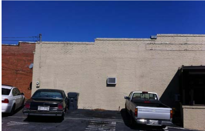
Here is an example of a historic stepped-back parapet wall, common on buildings in the Locust Grove commercial district to conceal gently sloping shed roofs.
