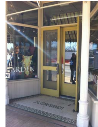
This Locust Grove historic storefront displays cast iron columns and historically appropriate glass.
