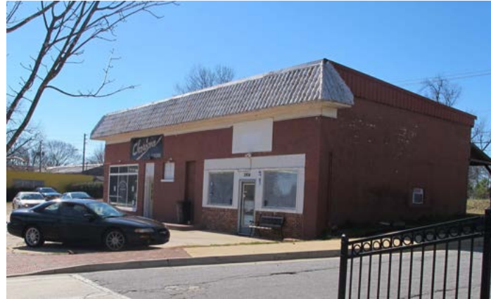
Like many other buildings in the Locust Grove historic commercial district, the structure located at 3904 Highway 42 has a horizontal emphasis due to its one story height and wide windows.
