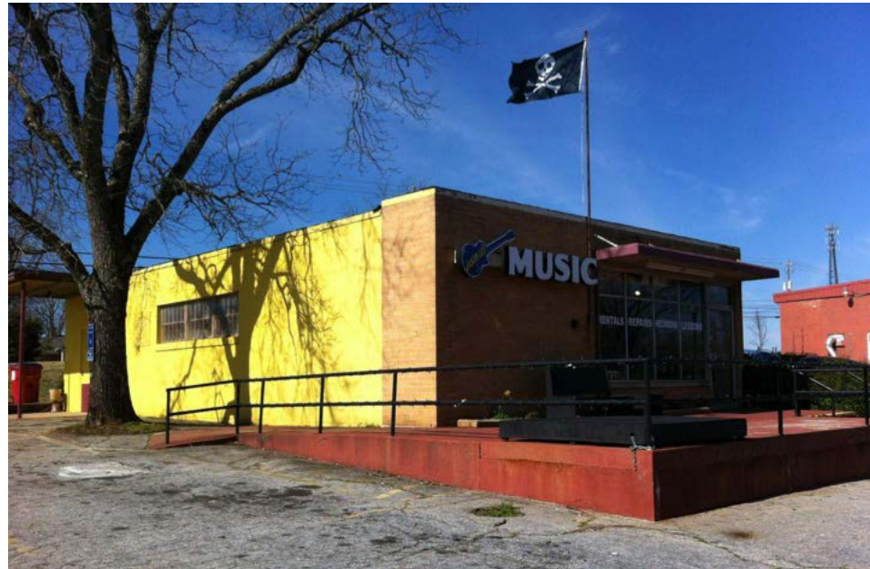
This former U.S. Post Office on U.S. Highway 23, just south of the commercial district, was built in the 1960s but displays International Style elements such as a flat roof, smooth surfaces, and simple windows set flush with the walls.
