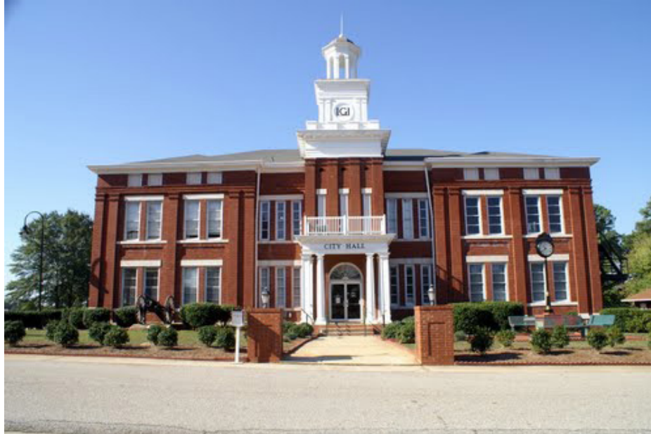
Locust Grove Institute as it stands today. It now serves as City Hall.
