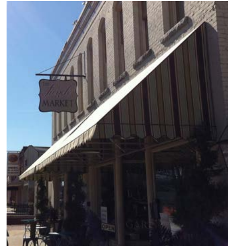
This awning is made of durable material and is installed at an appropriate height and location on the multistory building.
