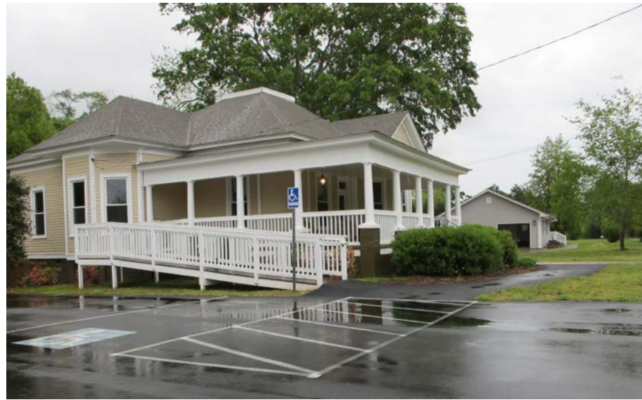
The location of ramps should be on the side or rear of a structure to have minimal visual impact.
