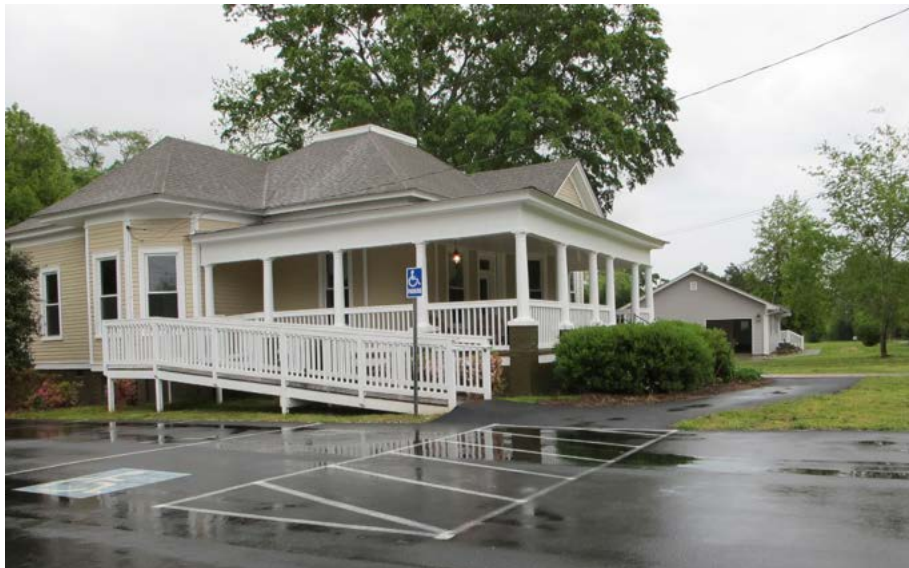
The location of ramps should be on the side or rear of a structure to have minimal visual impact.
