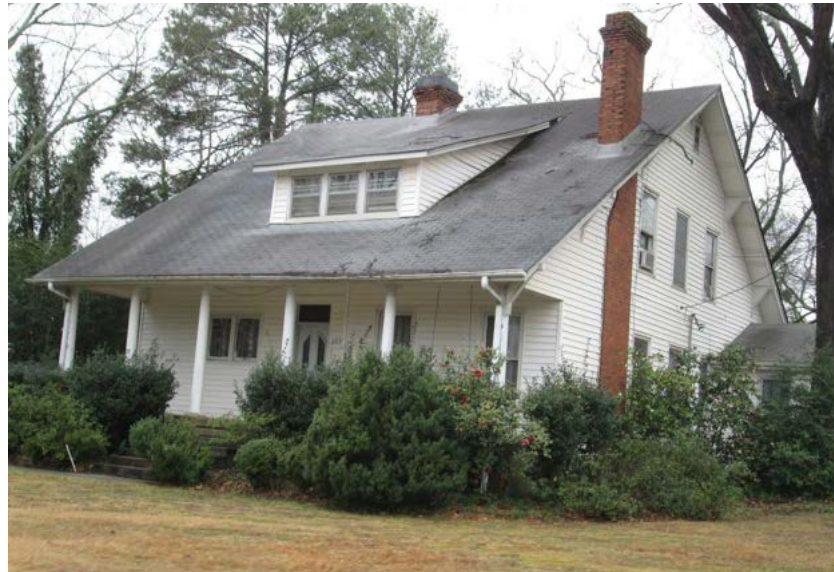
This is an example of a side gable Bungalow with a shed-roofed dormer, located on U.S. Highway 23. The porch has a wide overhang.
