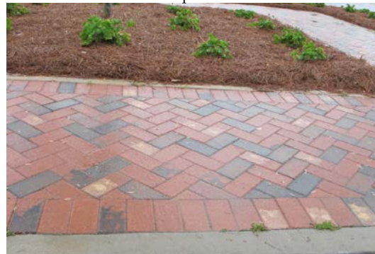
Brick pavers in a diagonal pattern are commonly found on the end of the commercial street blocks.
