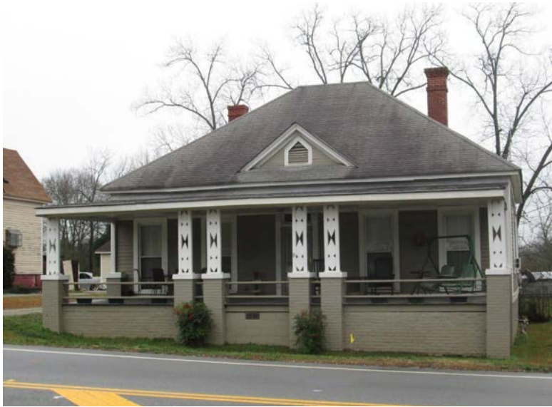
This example of a Pyramid Cottage on Peeksville Road is distinctive for its steeply pitched, symmetrical roof.
