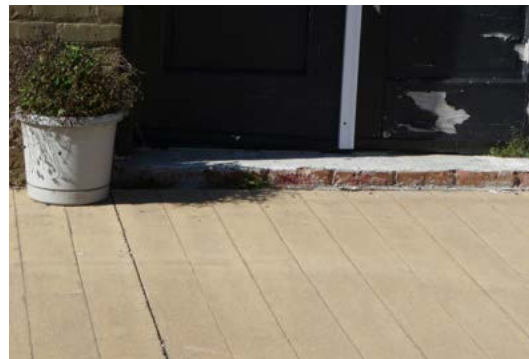
Concrete sidewalks designed to resemble wooden planks are the predominant style in the historic commercial district in Locust Grove.
