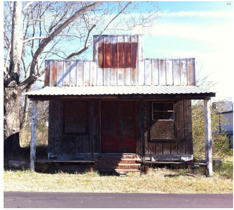
This historic Wood Frame Gable structure is on Jackson Street, across the railroad tracks, from the Locust Grove commercial district. Note the “general store” appearance with covered porch and front gable to display signage.
