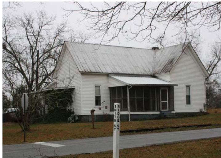
This Gabled Wing Cottage on Ridge Street has a gable front at one end, gabled roof, and a porch that covers the front door.
