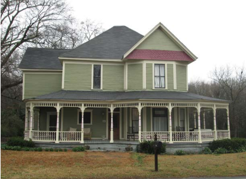
This two-story Queen Anne House on Peeksville Road has both front- and side-facing gables with a pyramidal roof in the center mass.
