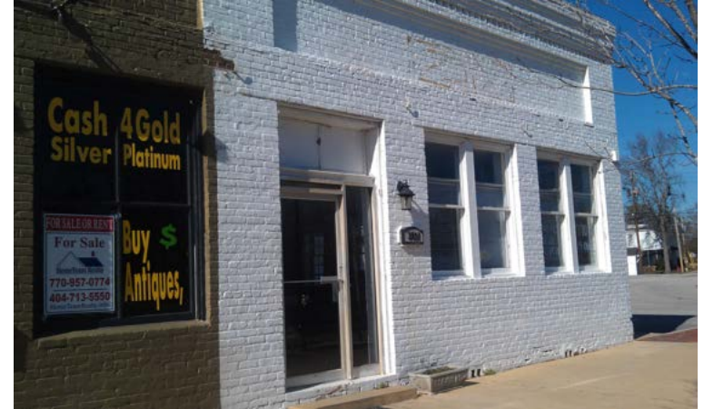
While painted, both 3831 and 3832 Highway 42 are constructed primarily of brick.
